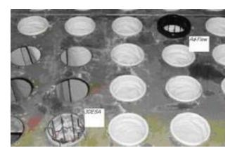
The Pic. 11. Montage of two types of filter bags
